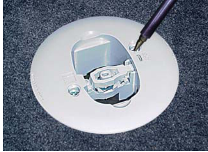
Step 2 Install carpet and secure the floor grommet into the floor, using a screwdriver to activate the inbuilt clamping mechanism.
